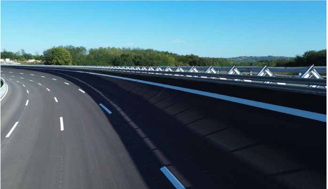
MEISER Road Safety vehicle restraint systems safeguard the demanding test tracks of AVL ZalaZONE
