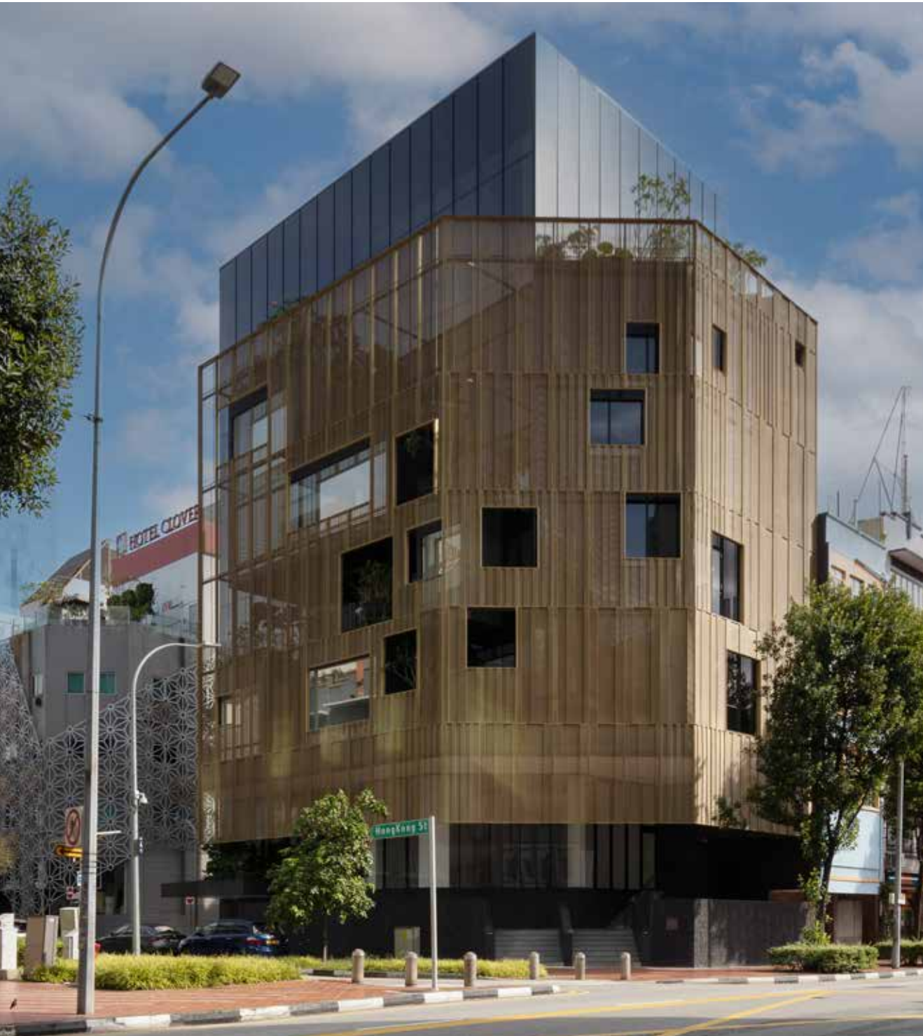
The Garden Curtain Wall in Singapore impresses with its continuous expanded metal façade, which lends the building a sense of lightness and transparency, as well as a striking architectural profile
