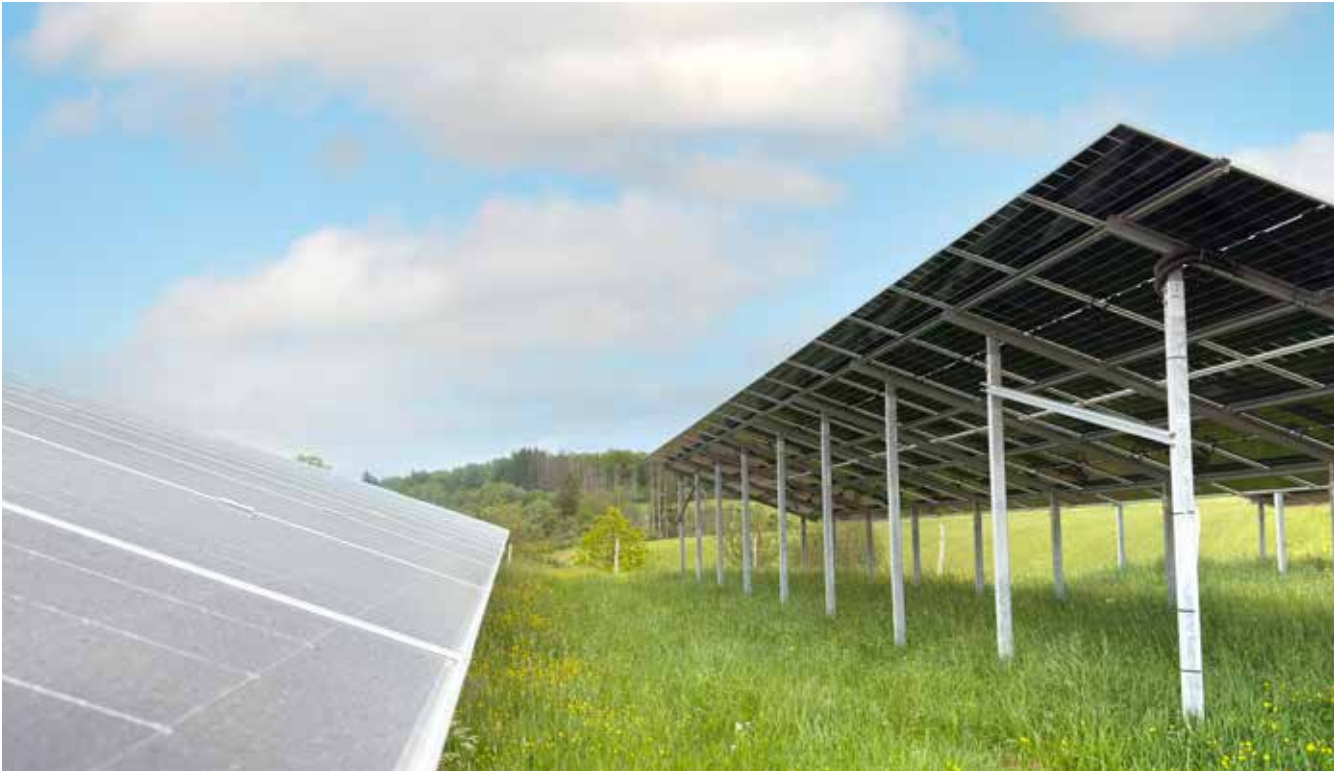
The two-pile MEISER Portrait mounting system in a solar park in Nonnweiler
